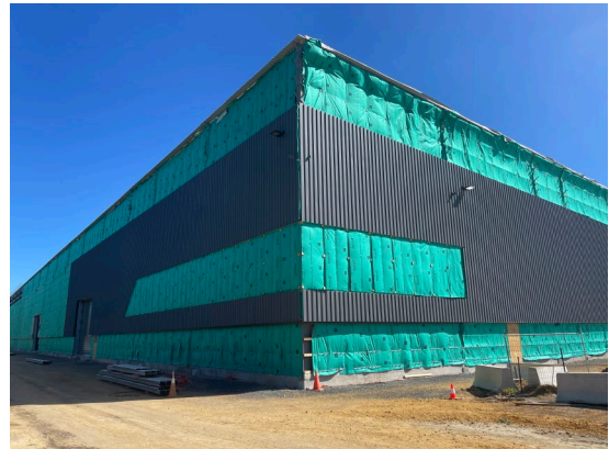
North-east corner of the NeXTimber manufacturing facility.
